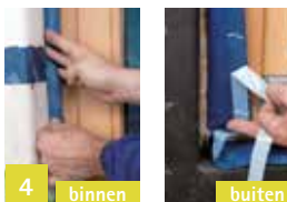
4 Band rondom in de dagkant vastkleven
