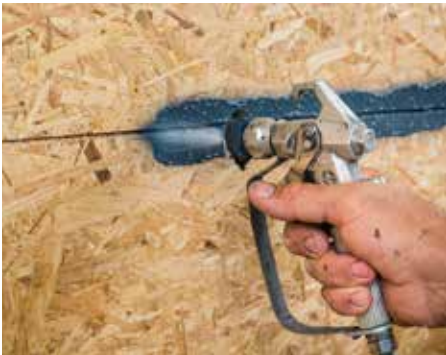
... joints between wood-based panels,
