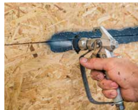
... joints between wood-based panels,
